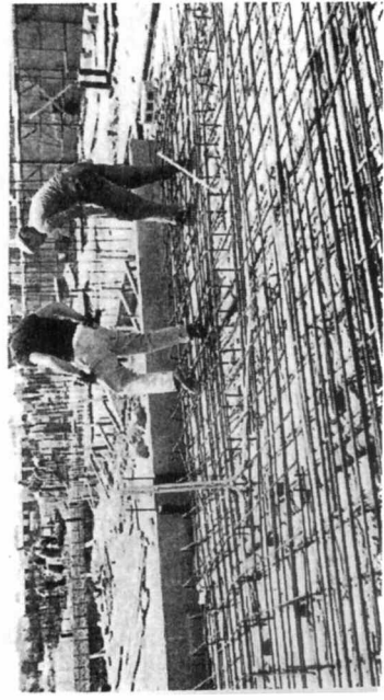
100 tons of steel rods have been placed into the slab, creating a strong unbreakable floor.
