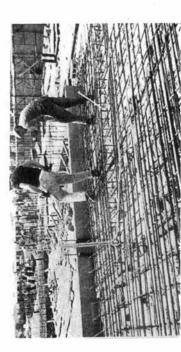
100 tons of steel rods have been placed into the slab, creating a strong unbreakable floor.
